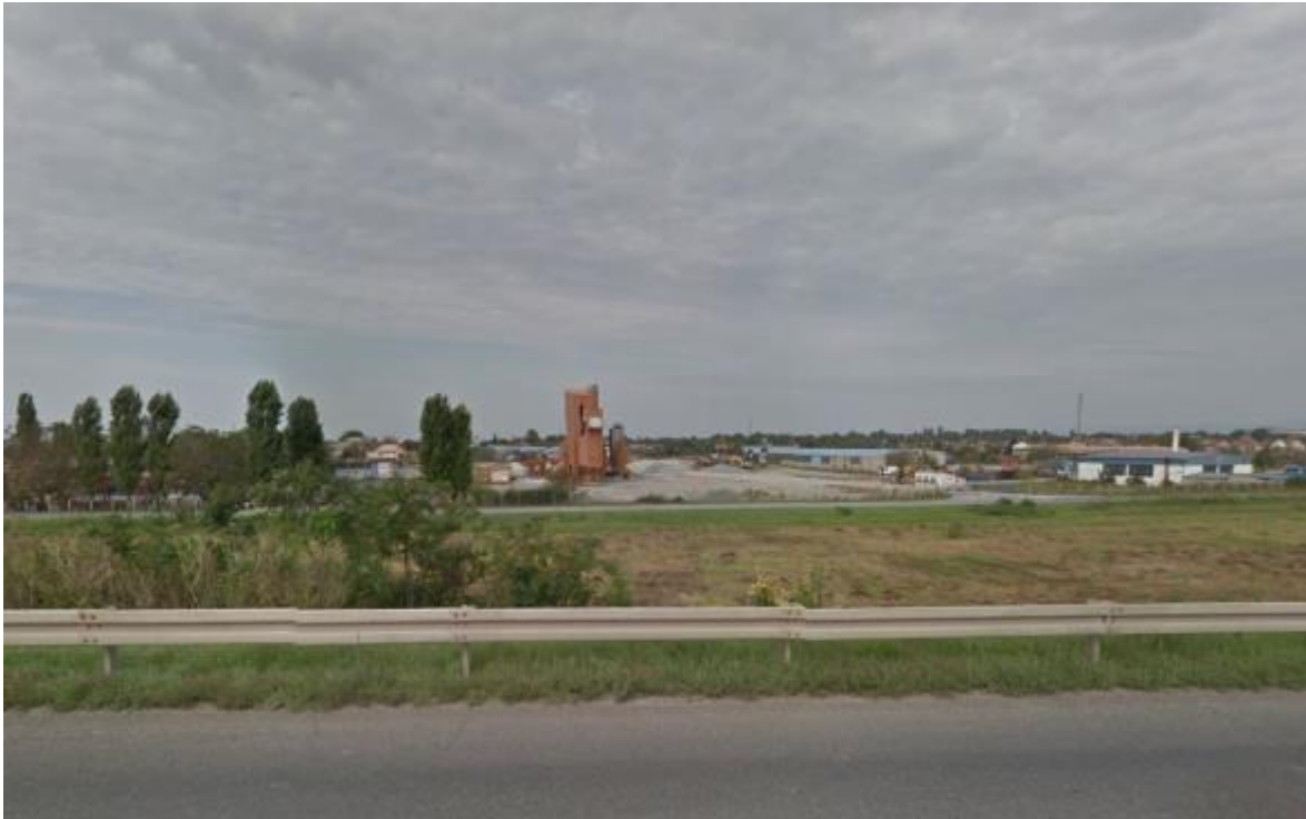
Picture 11 – Asphalt Plant “Borovica”
