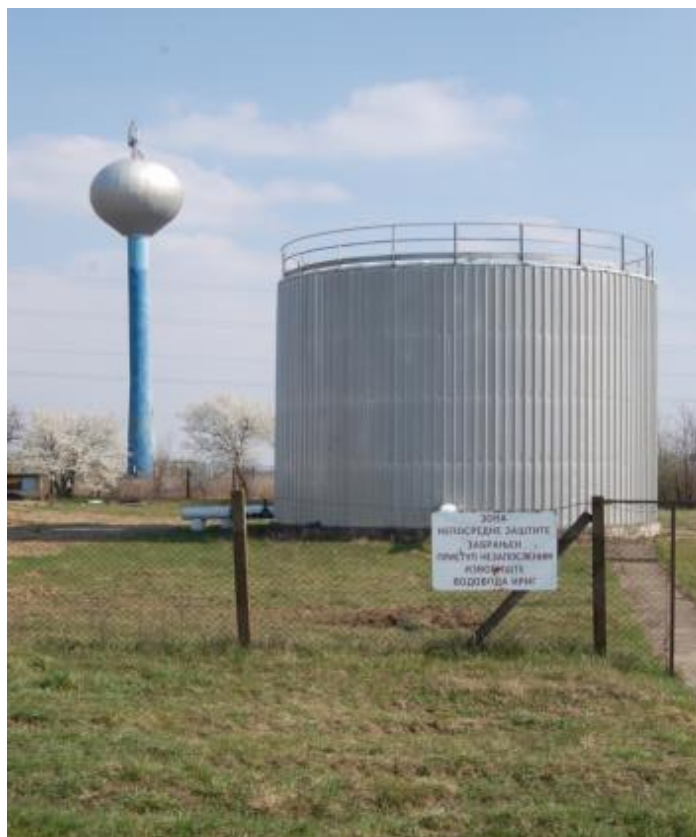
Picture 14 – Water reservoir
