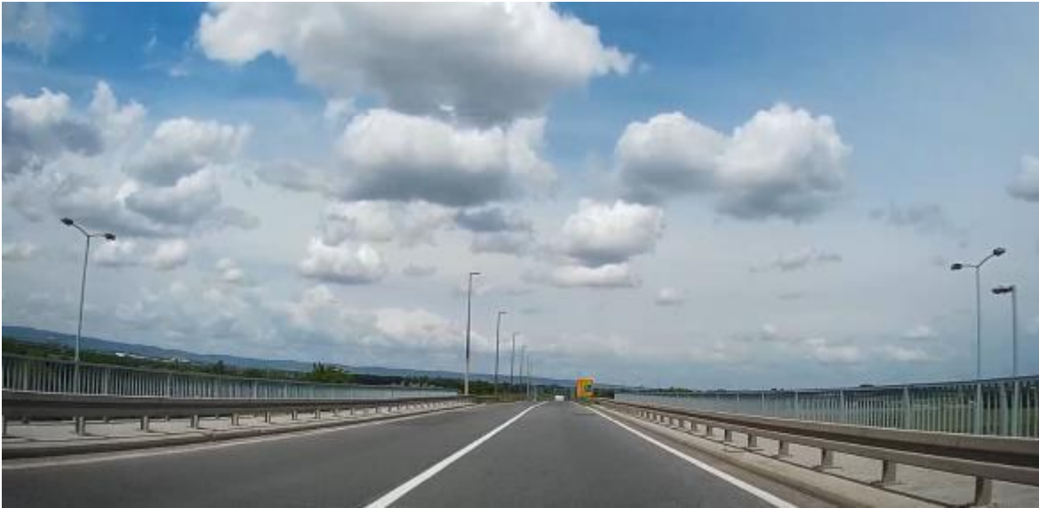
Picture 3 – Overpass on the motorway E 75 – end of the section
