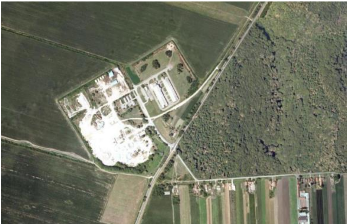
Picture 13 - „Galenika – Fitofarmacija“ and asphalt and concrete plant
