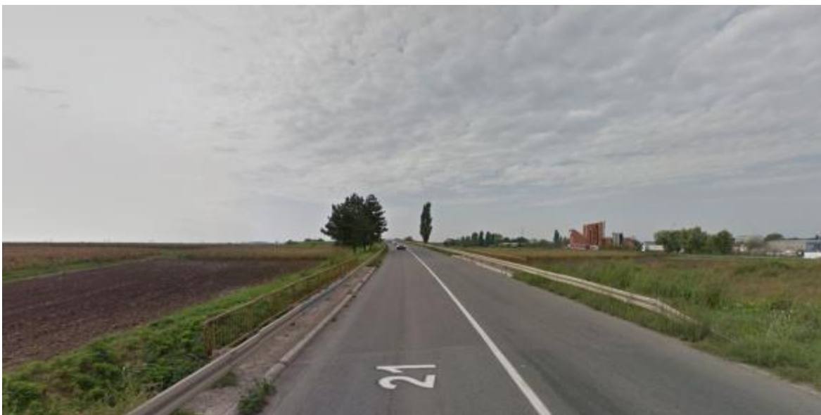
Picture 15 – Bridge on the Jelenački potok
