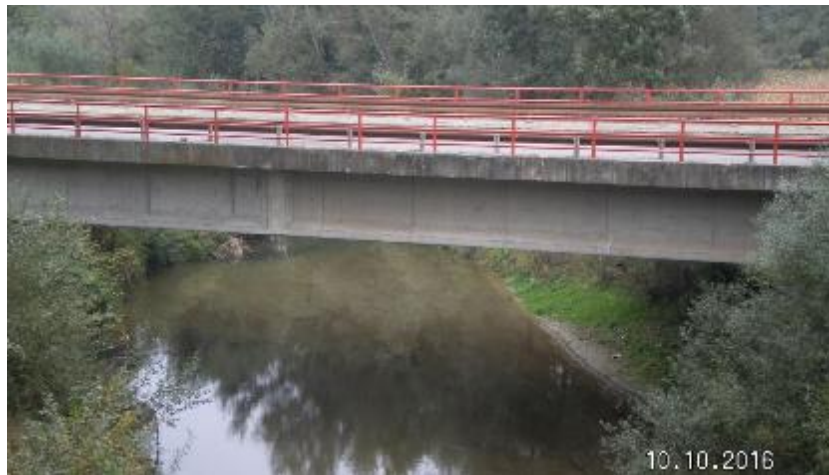
Picture 10. Bridge on the River Jasenica
