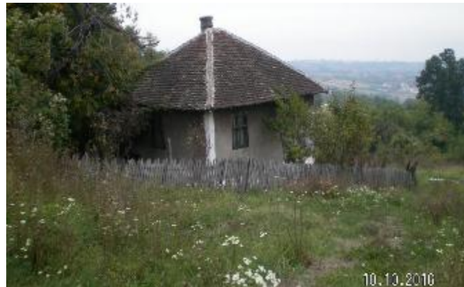
Picture 27. The building of the area of the existing landslides
