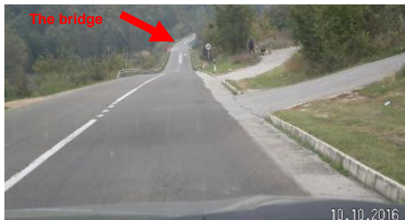
Picture 11. Surroundings the bridge on the river Jasenica
