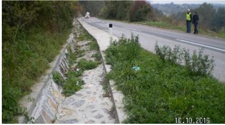
Picture 20. The existing drainage channel - Village Bozurnja
