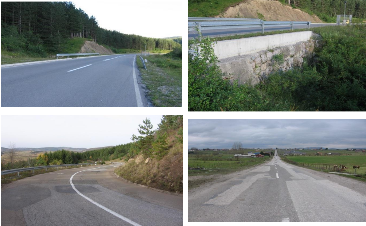
Picture 12: Typical segments along the section
