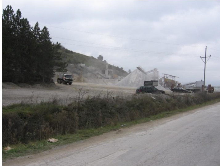
Picture 7: Quarry zone „ Wild River “ facilities for processing stone
