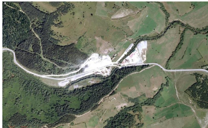
Picture 8: Quarry zone „ Wild River “ facilities for processing stone - location
