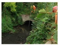
*Figure 5 Tubing \u03c62000mm at km 66+925*
