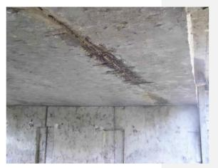
Figure 18 repair of the botom part of the pier
