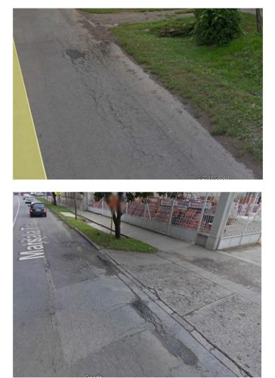
Figure 15. Example of damage of the road section
