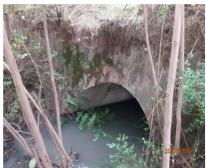
Figure 6 Solid-headed culvert at km 67+845
