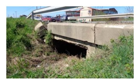
Picture 18. Box culvert for the occasional torrential watercourse
