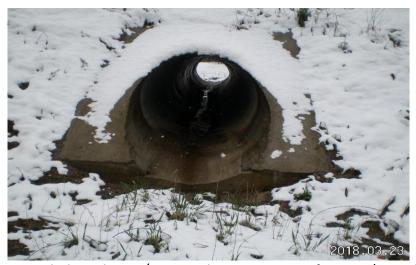
**Picture 13.** Tubular culvert Ø 1400 at km 10+337 − no function/ out of order
