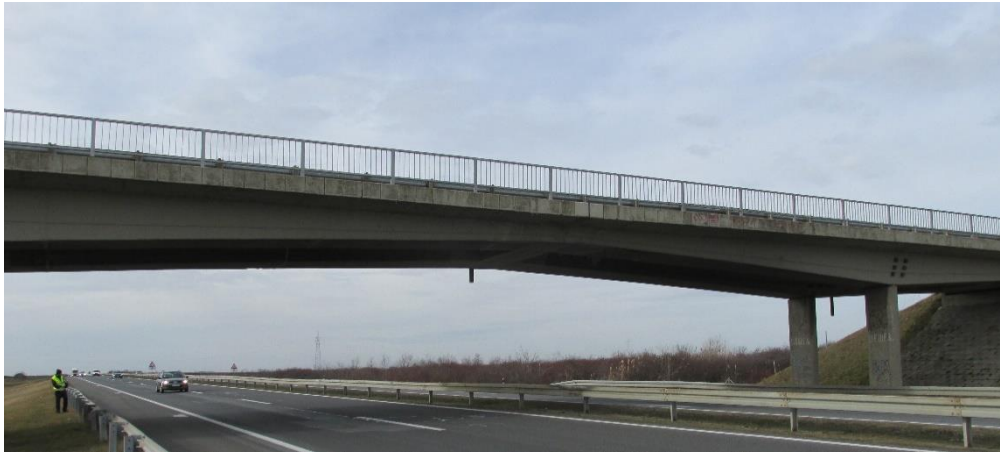
Figure 24. Overpass at km 65+320
