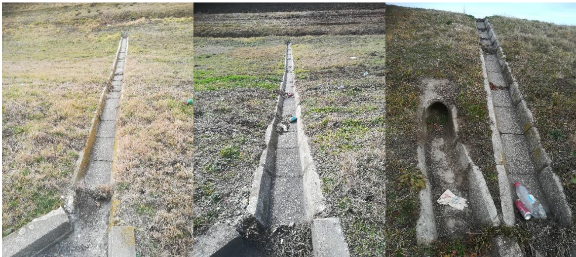
Figure 13. The flumes on the subject section
