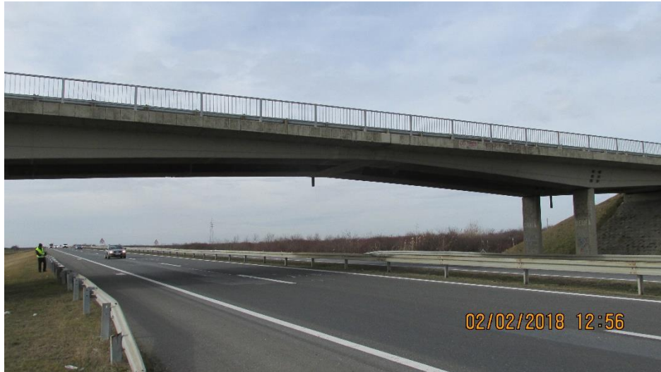
Figure 10. Overpass at km 65+320
