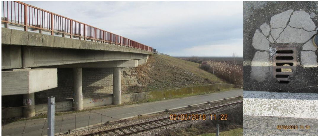
Figure 17. Overpass across the railroad Ruma - Sabac at km 60+752
