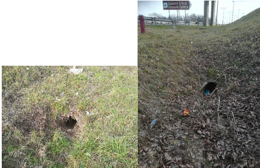
Figure 22. Pipe culvert at km 57+300
