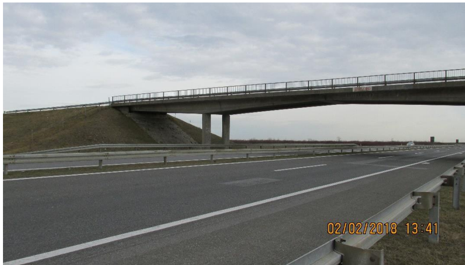
Figure 11. Overpass at km 68+200
