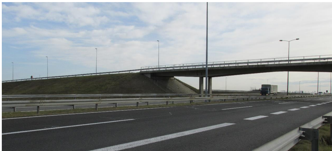
Figure 23. Overpass at km 57+850
