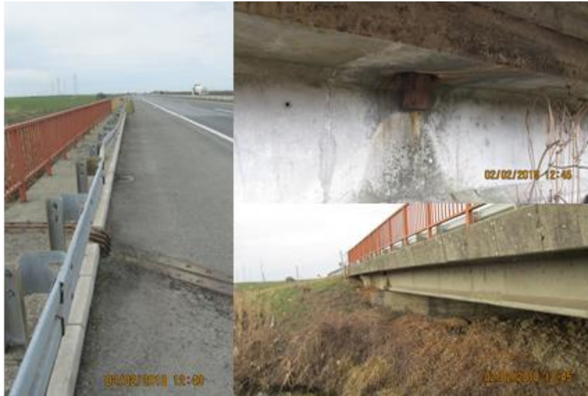
Figure 8. The bridge across the canal Jarcina at km 65+040.00
