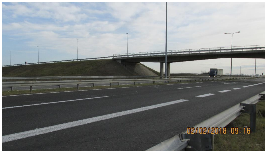
Figure 9. Overpass at km 57+850
