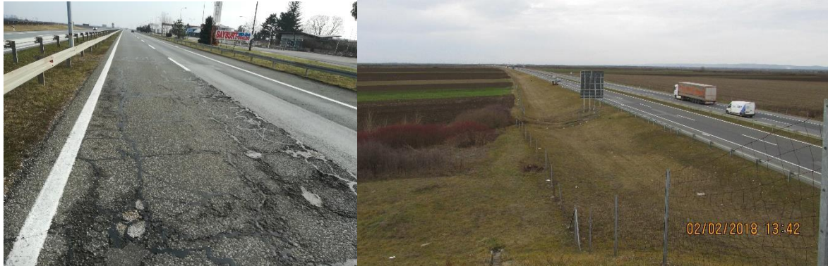
Figure 6. Typical parts of the subject section
