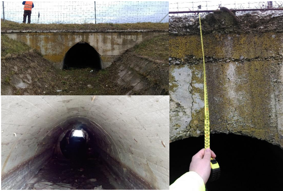
Figure 20. Arched culvert at km 57+355
