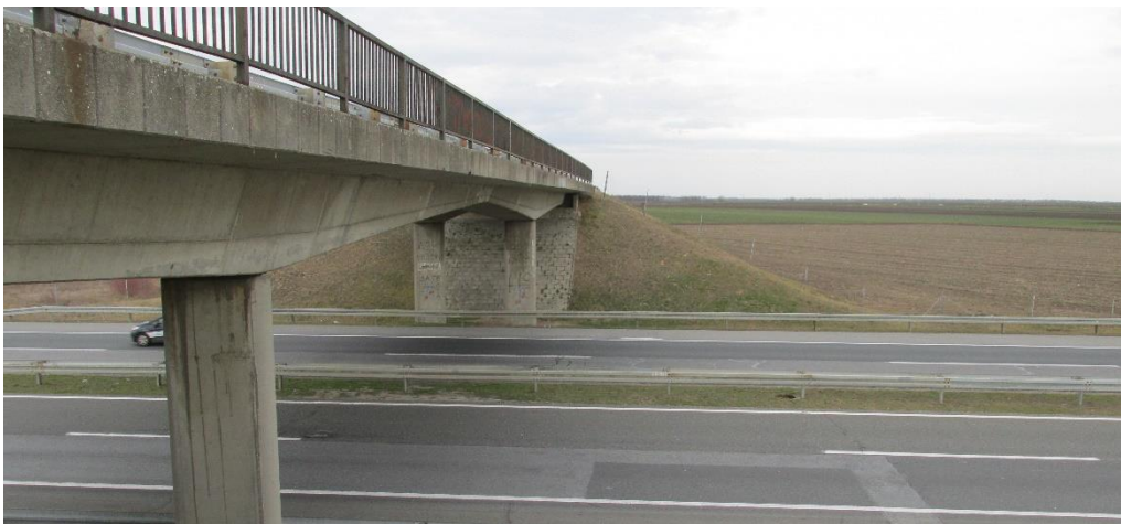
Figure 25. Overpass at km 68+200
