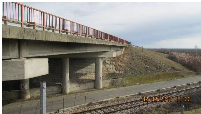
Figure 7. An overpass over the railroad Ruma - Sabac at km 60+752
