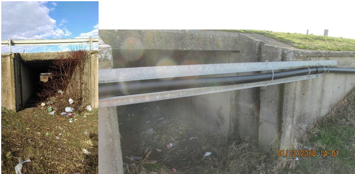
Figure 21. Box culvert at km 66+025
