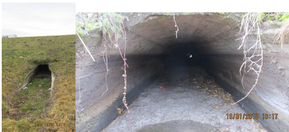
Figure 24 Arched culvert at km 47+874
