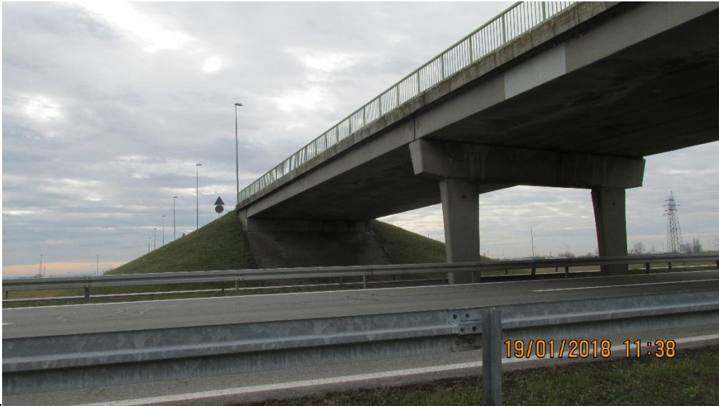
Figure 27 Overpass at km 44+220
