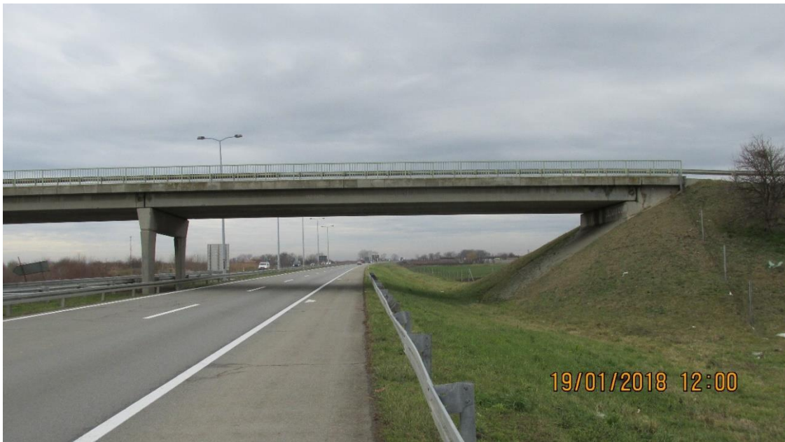
Figure 11 Overpass at km 43+550
