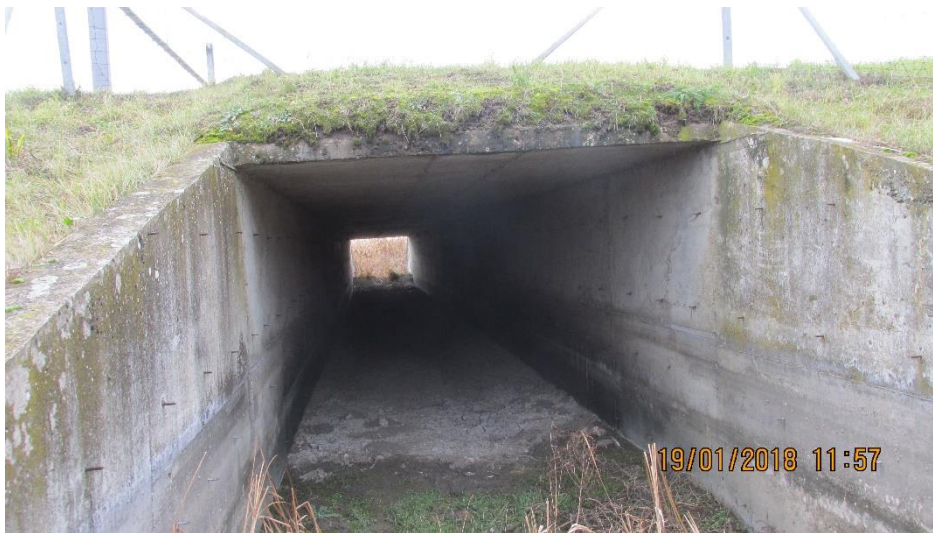
Figure 23 Slab culvert at km 43+867
