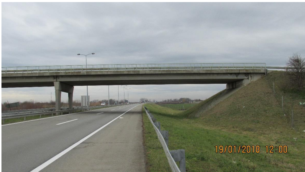
Figure 26 Overpass at km 43+ 550
