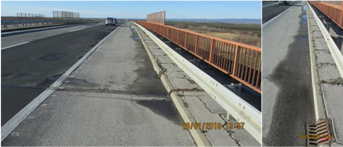
Figure 8 Voganj Overpass at km 49+250
