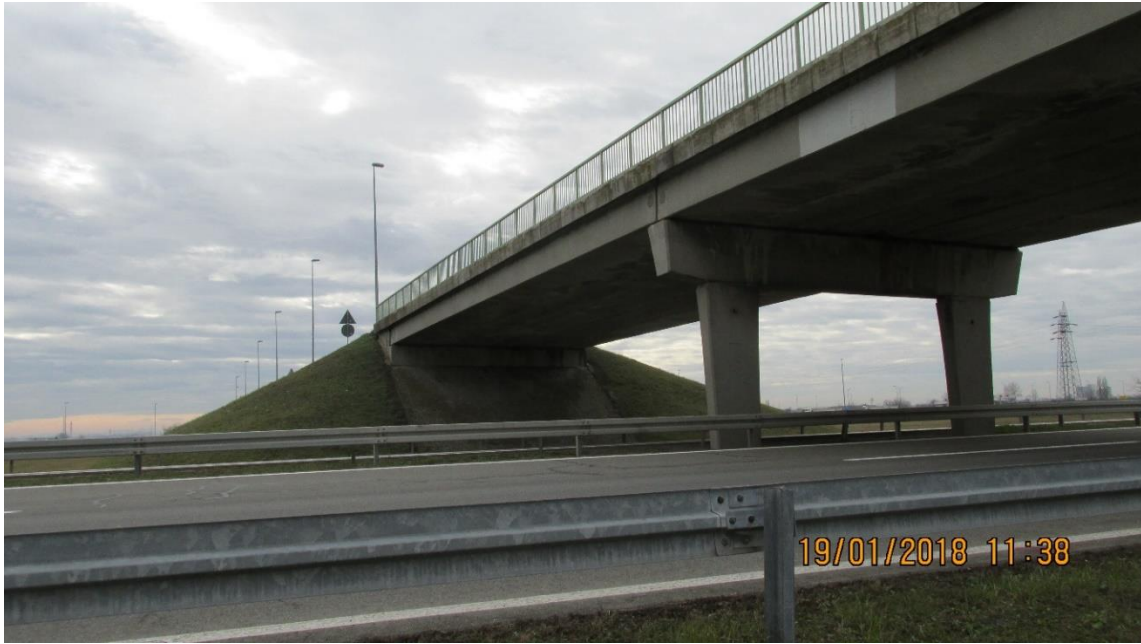
Figure 12 Overpass at km 44+200
