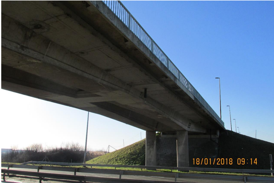
Figure 14 Overpass at km 57+313
