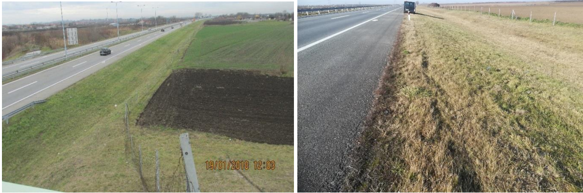
Figure 6 Typical parts of the subject section
