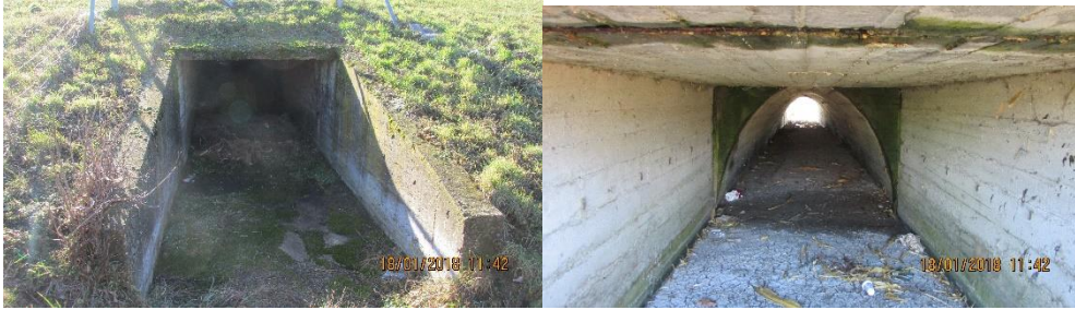
Figure 25 Combined culvert at km 53+430
