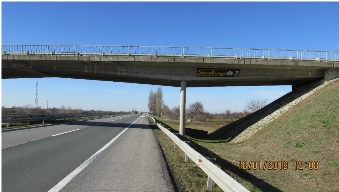
Figure 13 Overpass at km 52+684
