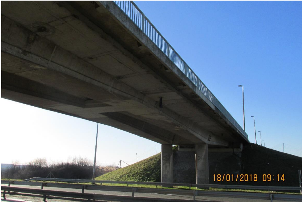
Figure 29 Overpass at km 57+313
