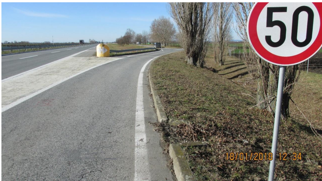
Figure 18 Rest area at km 52+250
