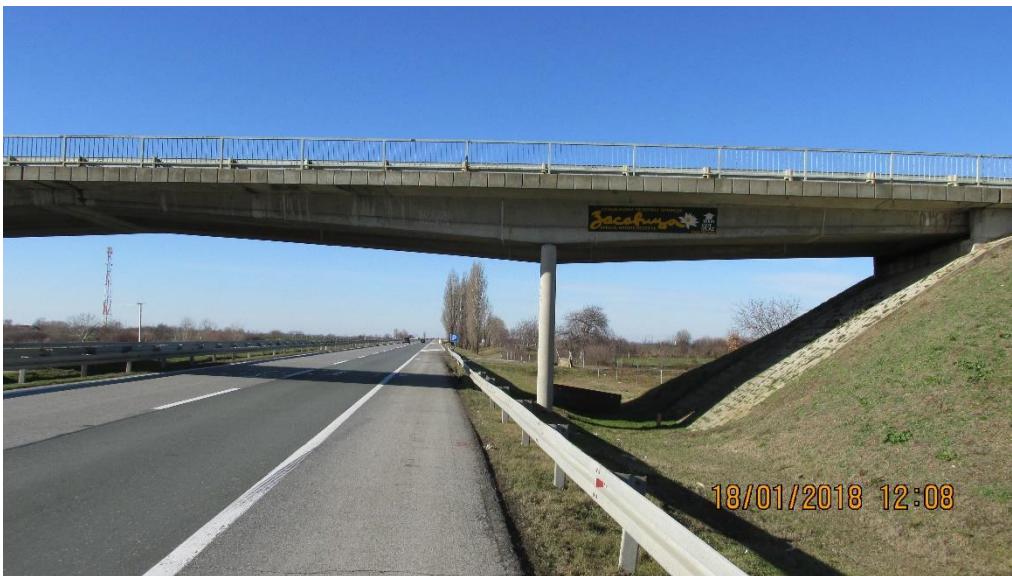
Figure 28 Overpass at km 52+684
