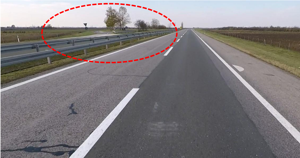
Figure 17 Rest area at km 51+300
