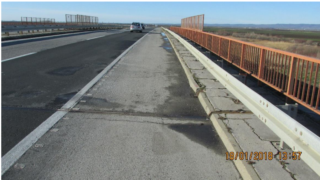
Figure 19 Voganj overpass at the chainage of km 49+243.
