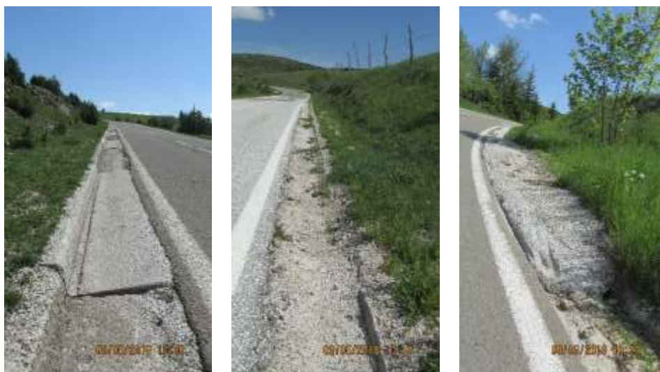
Figure 6. Gutters on the observed road section
