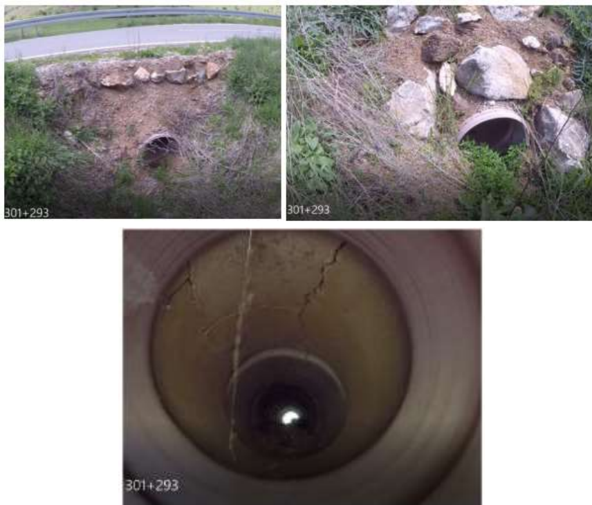
Figure 189. The pipe culvert at km 301+293
