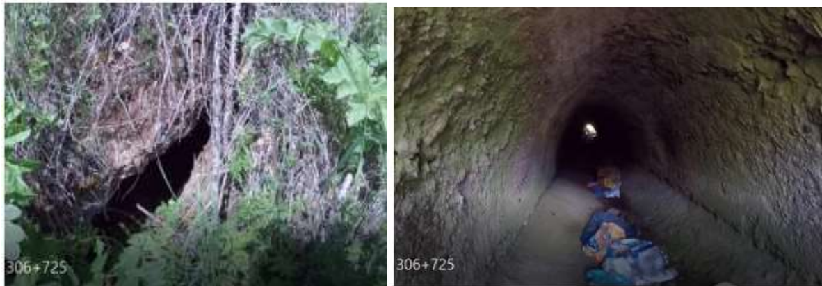
Figure 178. The arched culvert at km 306+725
