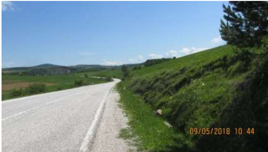
Figure 7. Canal on the observed road section
