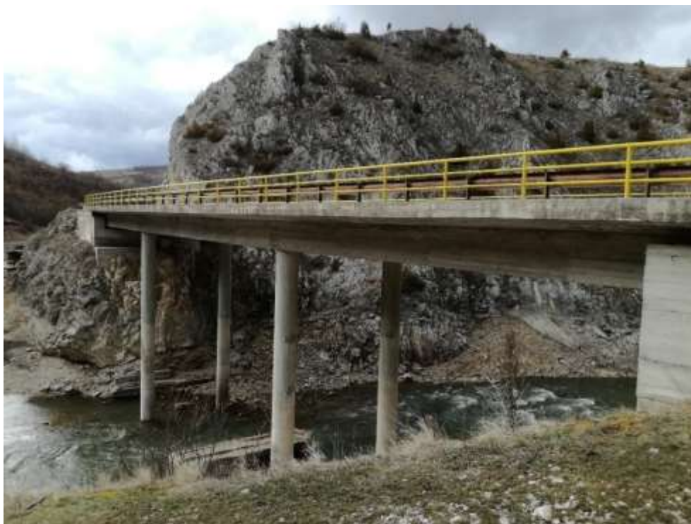
Figure 167. The Bridge over the Vapa River at km 305+350
