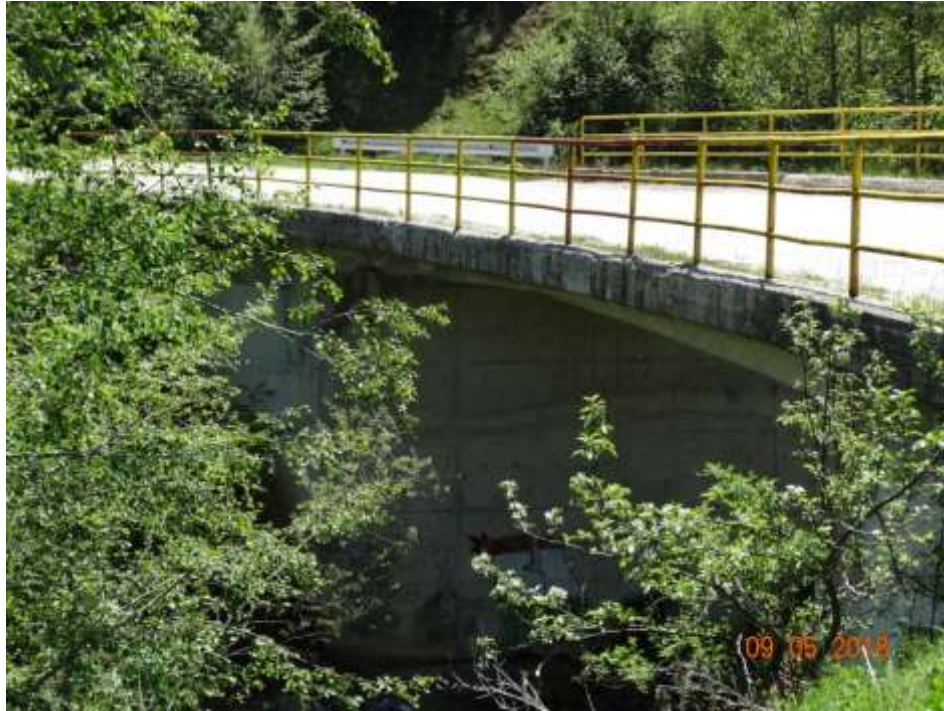
Figure 156. The Bridge over the Kladnica River at km 292+810
