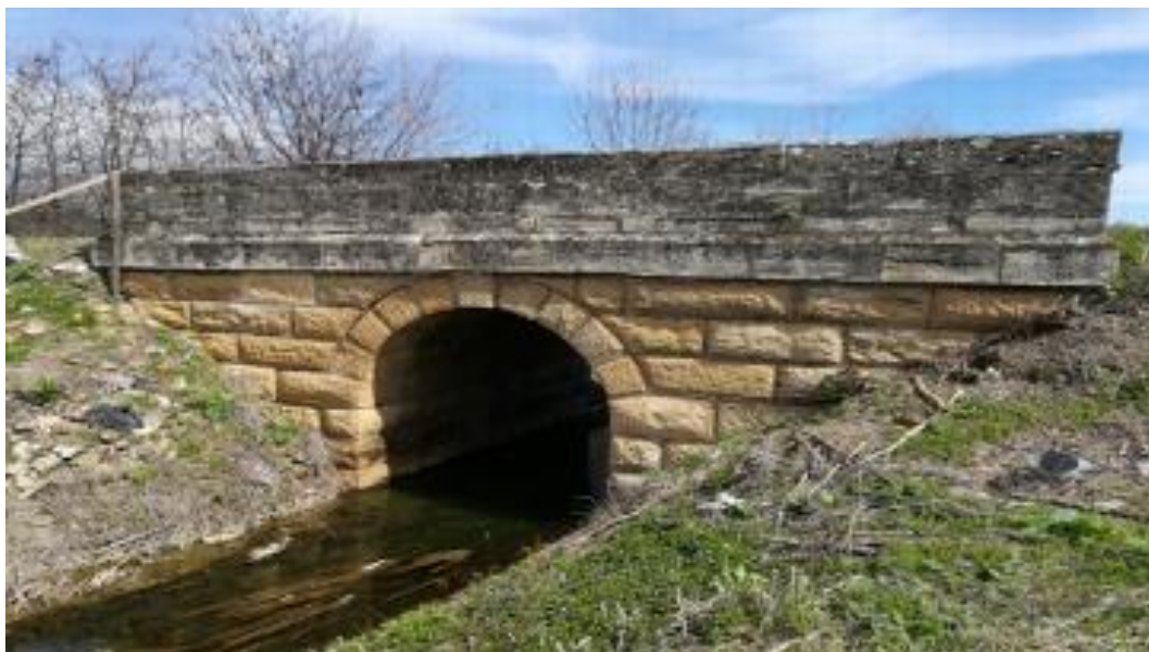
Figure 11. Culvert over Canal of tribute to Jasenicka River
