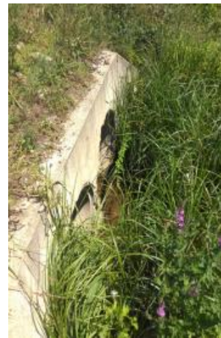
Figure 8. Culvert \phi 1000 at km 190+106.43
