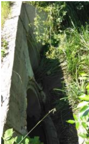
Figure 7. Culvert \phi 1000 at km 190+106.43
