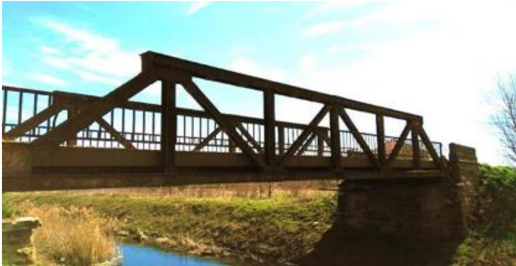
Figure 9. The bridge over Jasenicka River
