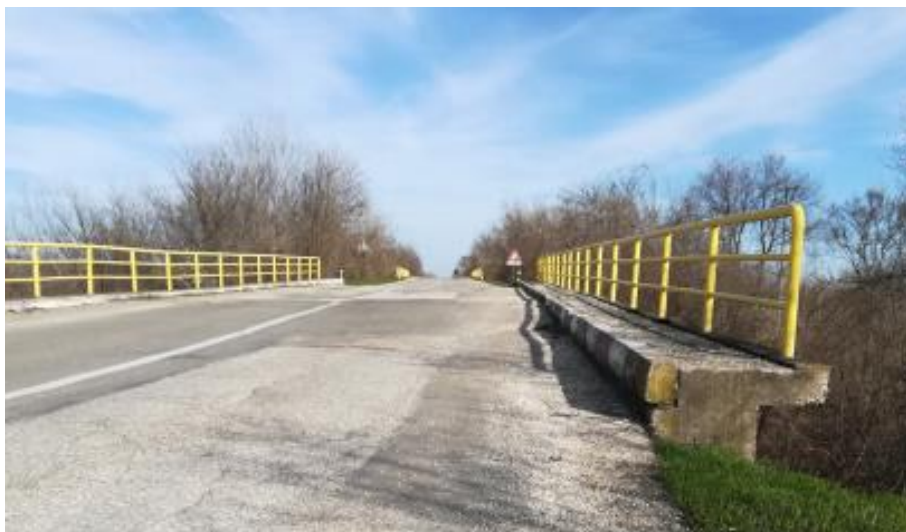
Figure 13. The bridge over Sikolska River
