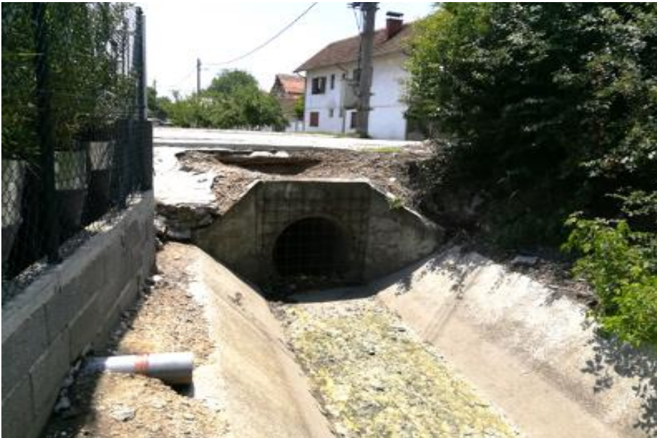
Figure 6. Negotin – crossing with concrete canal
