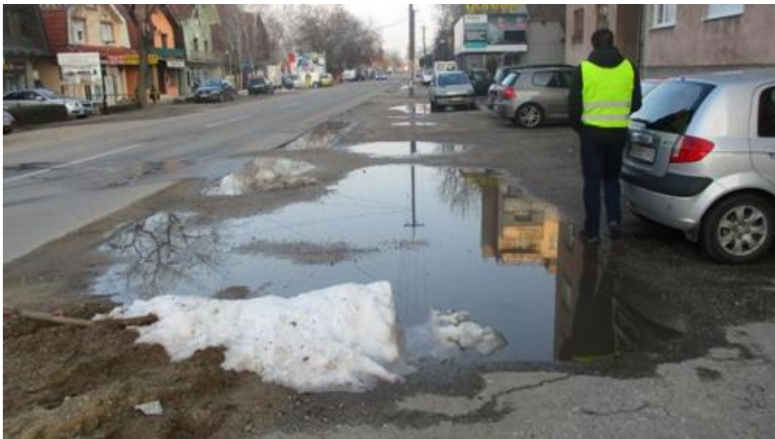
Figure 4. Negotin – part of the road across the concrete canal
