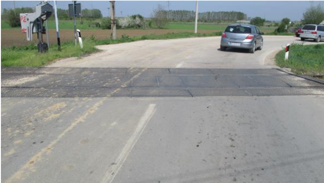
Figure 18. Reconstructed railway crossing at km 188+670
