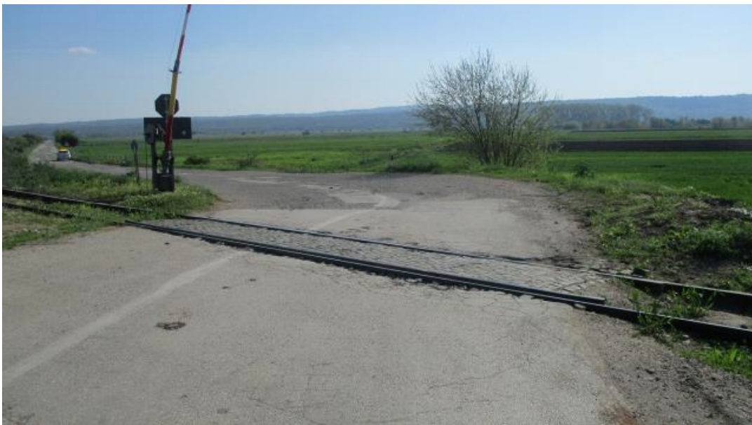
Figure 19. Railway crossing at km 194+896
