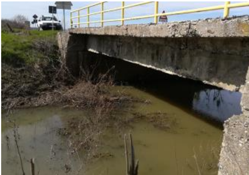
Figure 12. Structure over canal "Drain barrier"
