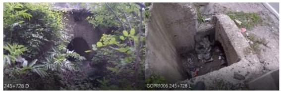
Figure 25. The arched culvert at km 245+728, outlet and inlet structure of the culvert
