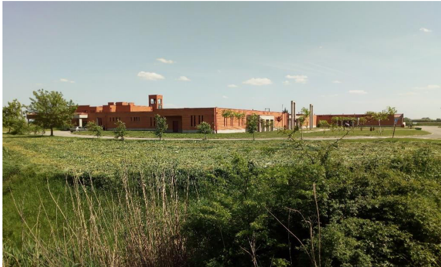
Figure 17. Parking lot in front of a new cemetery at ~ km 125+250
