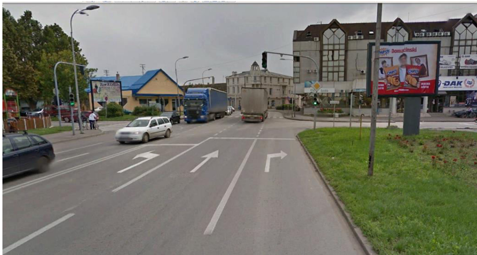
Figure 4. The beginning of the road section
