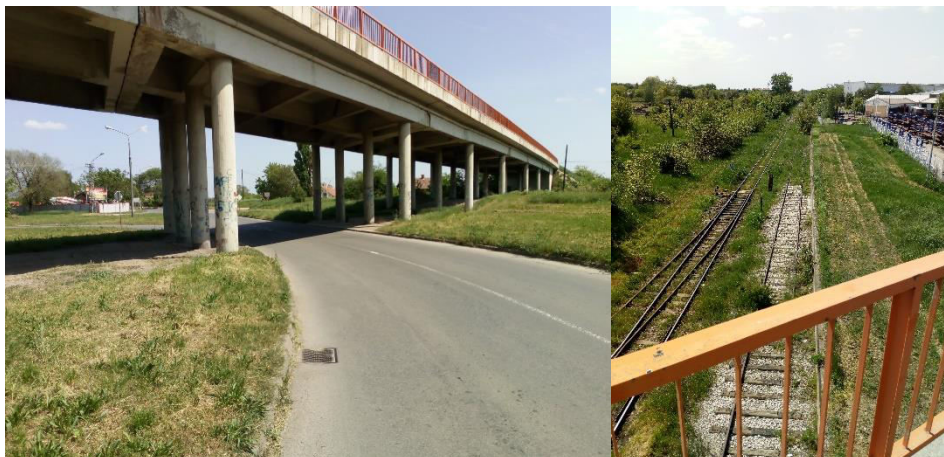
Figure 20. Bekov overpass at ~ km 124+060
