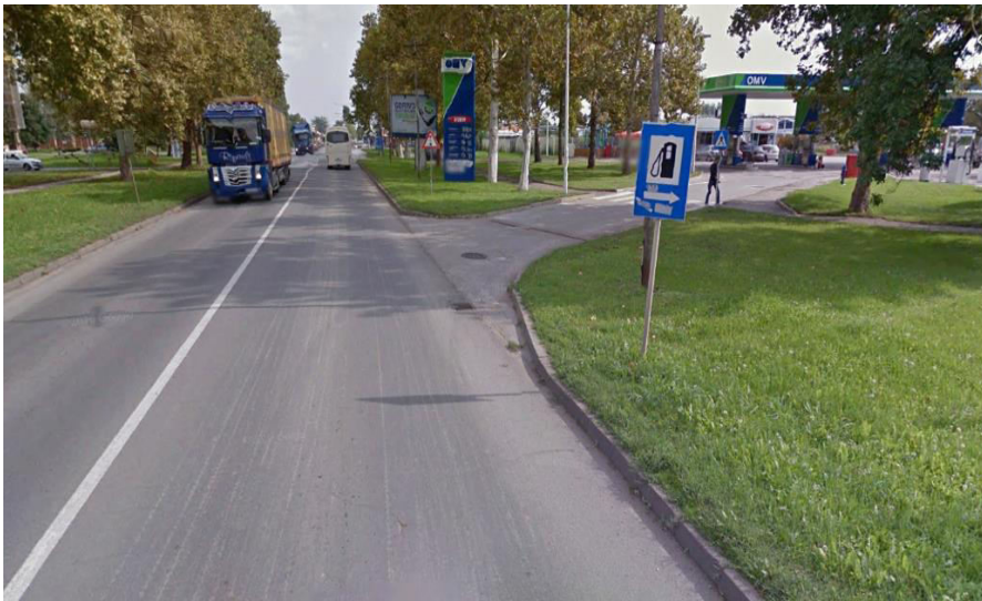
Figure 15. Petrol station „OMV” at ~ km 123+400
