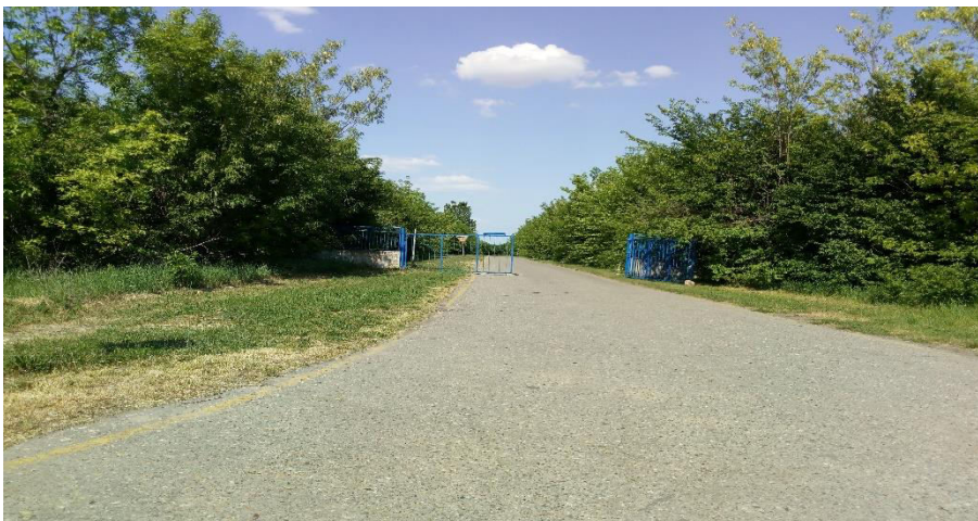
Figure 19. Airport at ~ km 129+420
