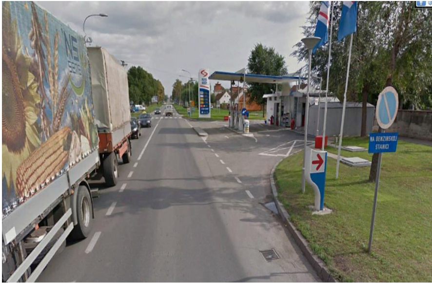
Figure 14. Petrol station „NIS” at ~ km 123+125
