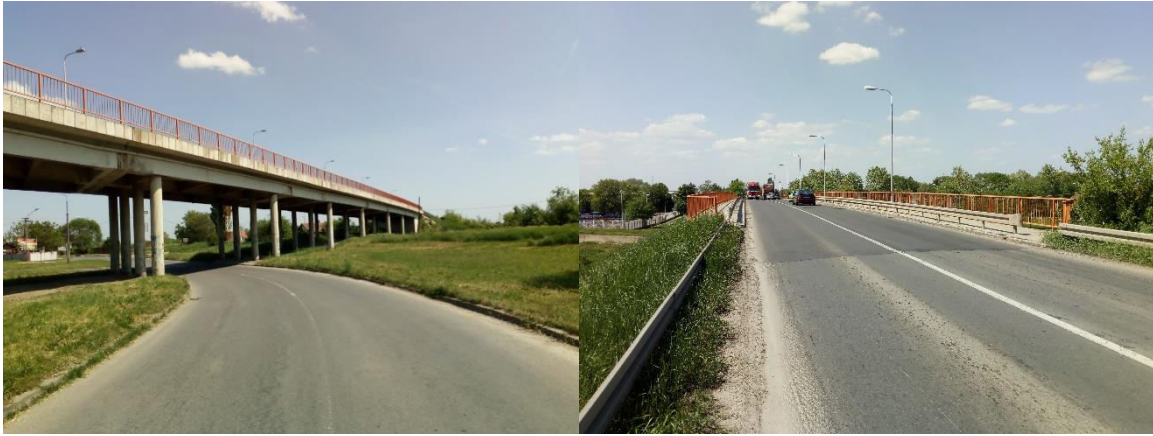
Figure 2. Bekov Overpass at ~ km 124+060
