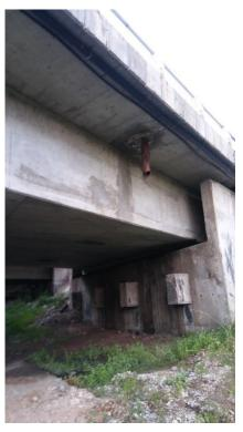
Figure 16. The bridge drains
