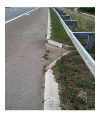
Figure 17. Drainage with a curb system and drainage cocrete gutters in front and behind the bridge
