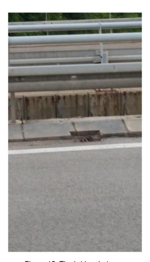
Figure 15. The bridge drains
