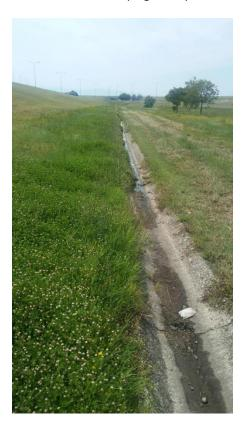
Figure 4. Ditch with concrete cover
