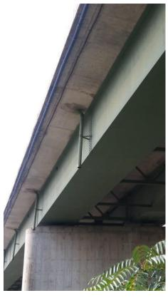
Figure 18 and 19. The bridge drains
