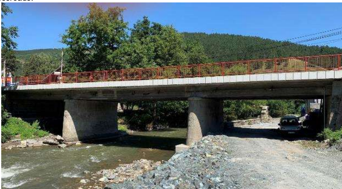
Pictures 3: Bridge over the river Studenica in Ušće (station km 203 + 700)
