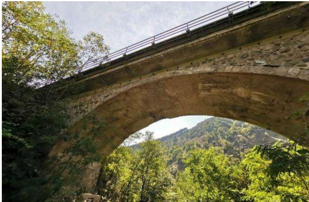
Pictures 5 and 6: Bridge over the river Gokcanica (station km 209 + 039)
