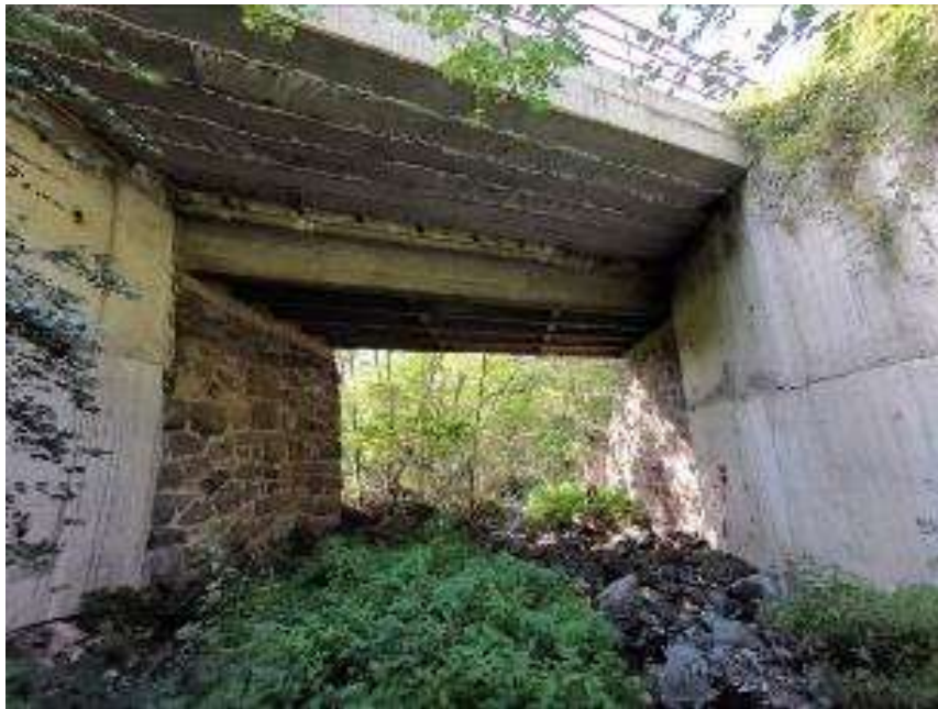
Pictures 8: Bridge over the Markovska river (stat. km 212 + 229)
