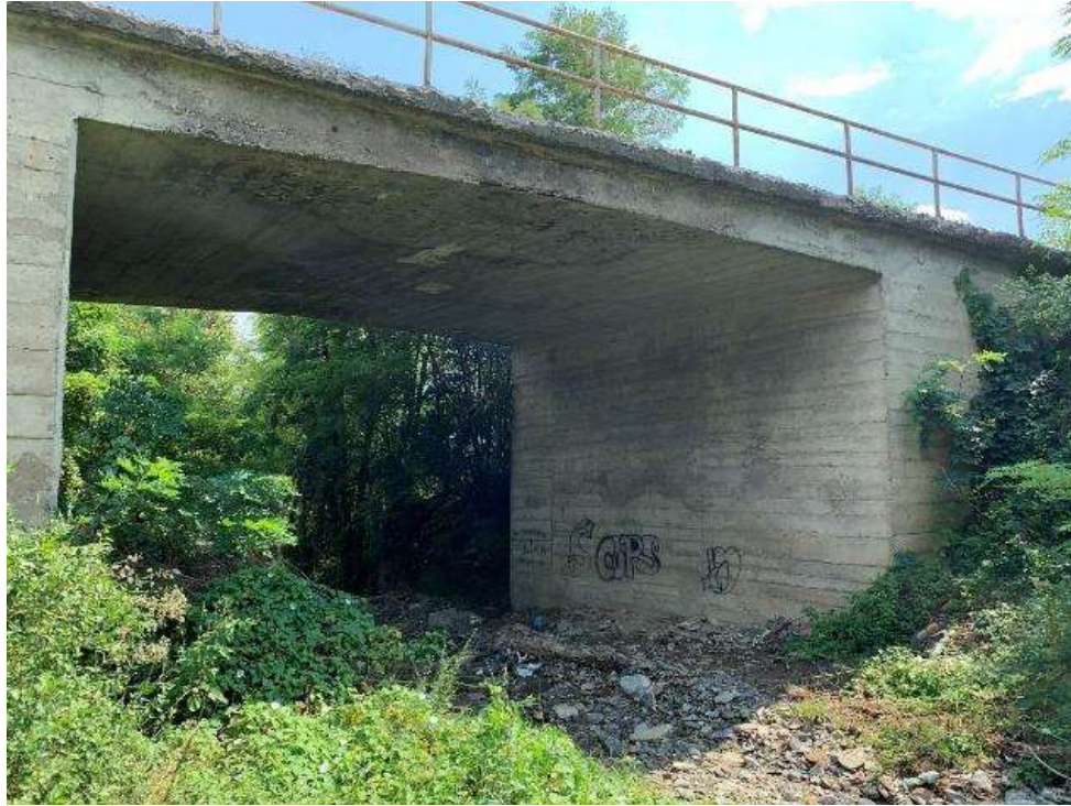
Pictures 13: Bridge over the stream in Baljevac (stat. km 222 + 184)
