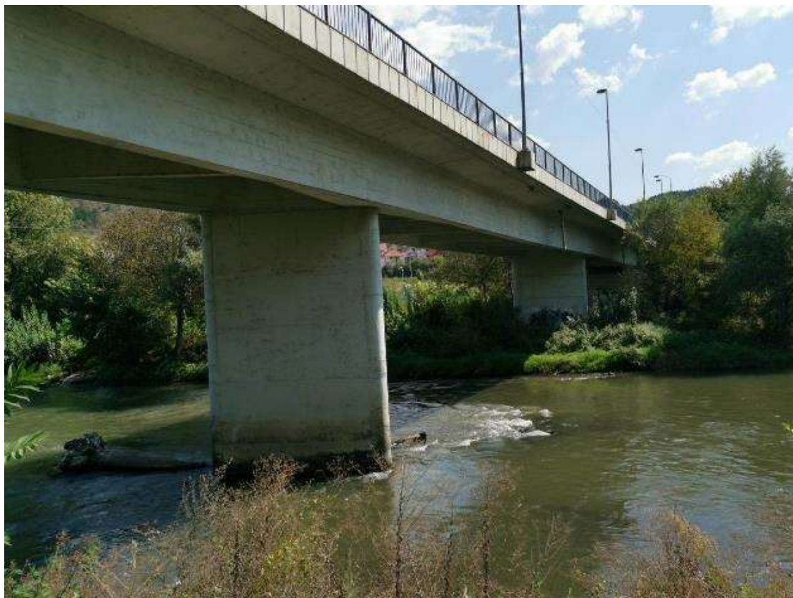
Pictures 15: Bridge over the river Ibar in Raska (stat. km 234+742.27)
