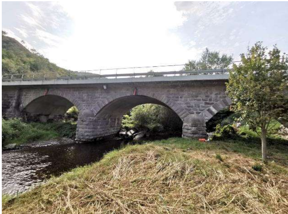
Pictures 14: Bridge over the river Brevnica (stat. km 226 + 760)
