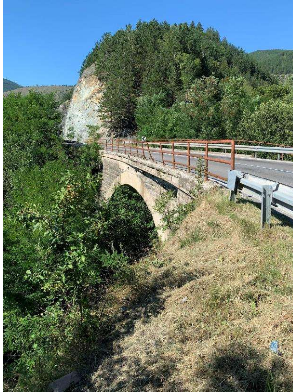
Pictures 7: Bridge over the stream in Bare (stat km 210 + 638)
