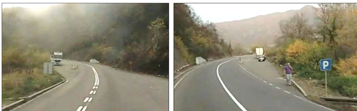
Pictures 34: Built parking lot next to the state road, stationing km 218 + 875.00
