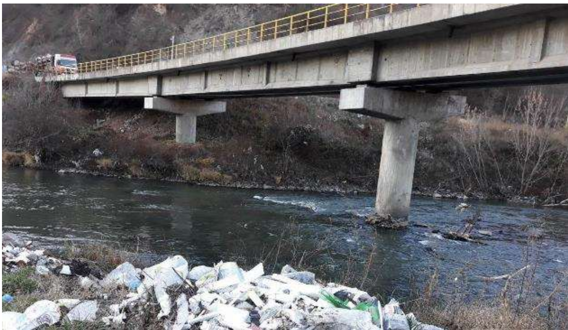
Pictures 10: Bridge over river Ibar in Biljanovac (stat. km 218 + 711)
