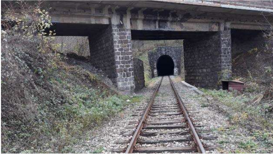
Pictures 9: Bridge over the railway in Bojanici (station km 213 + 194)
