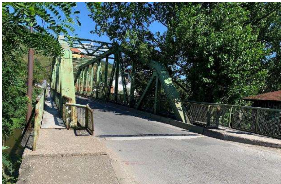
Pictures 4: Bridge over the river Ibar in Ušće (station km 203 + 960)
