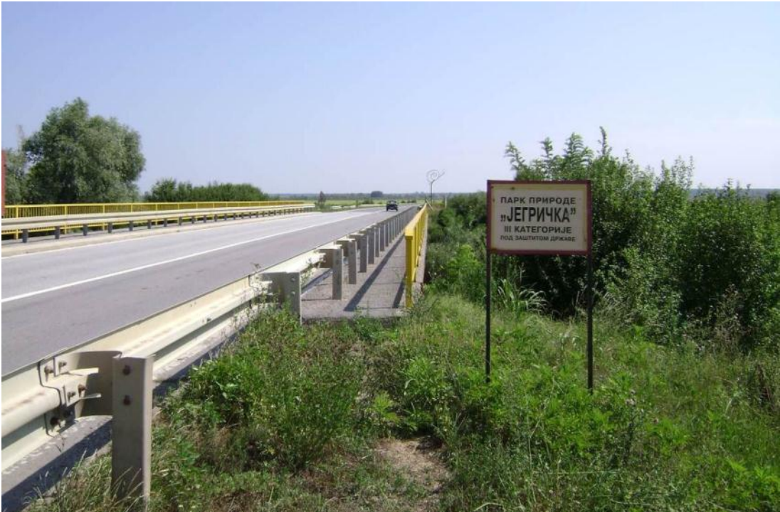
Figure 3.13: Bridge over Jegricka Canal and information about protected area
