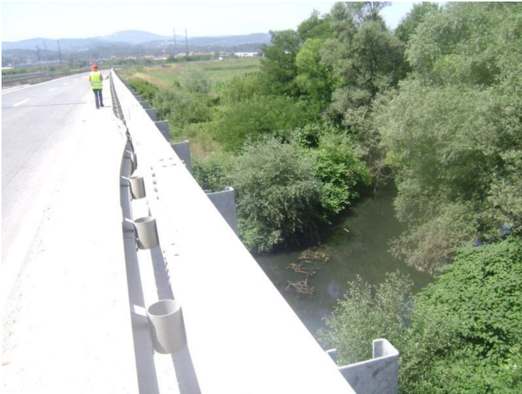
Figure 3.3: Bridge over Skrapez River
