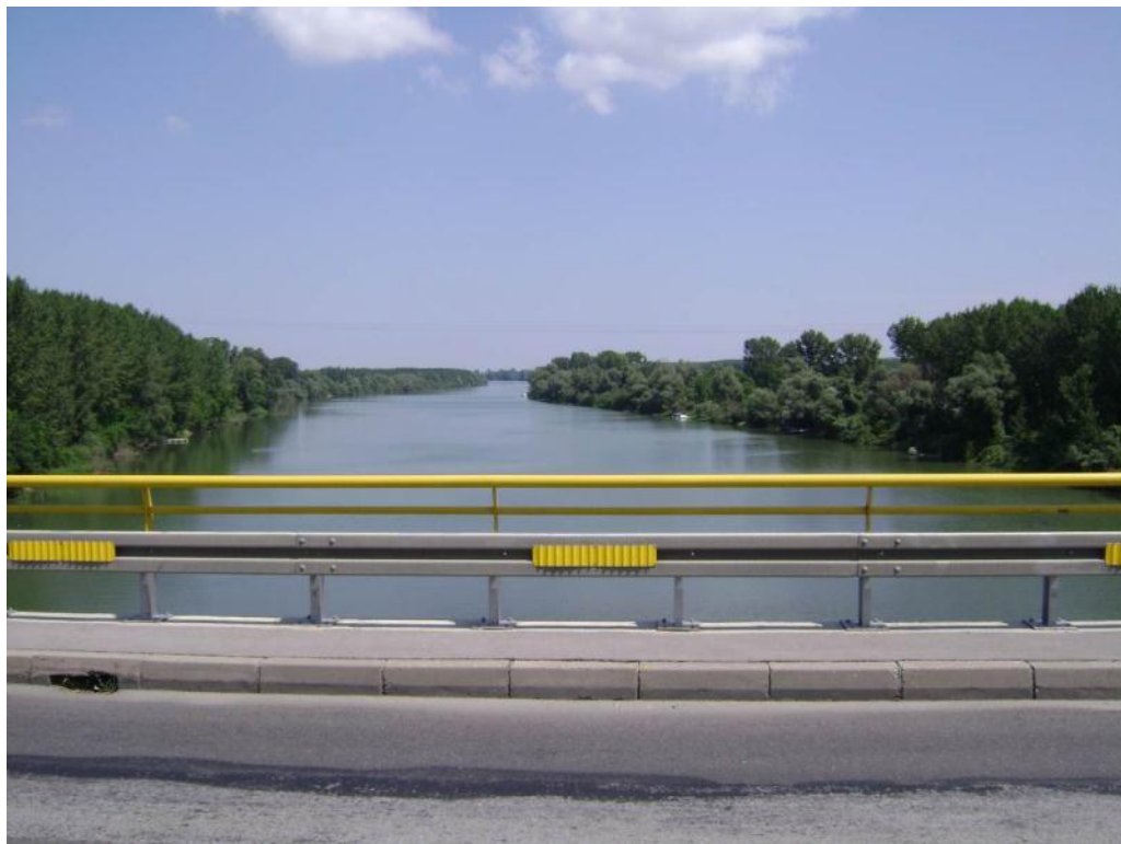
Figure 3.11: Bridge over Tisa River
