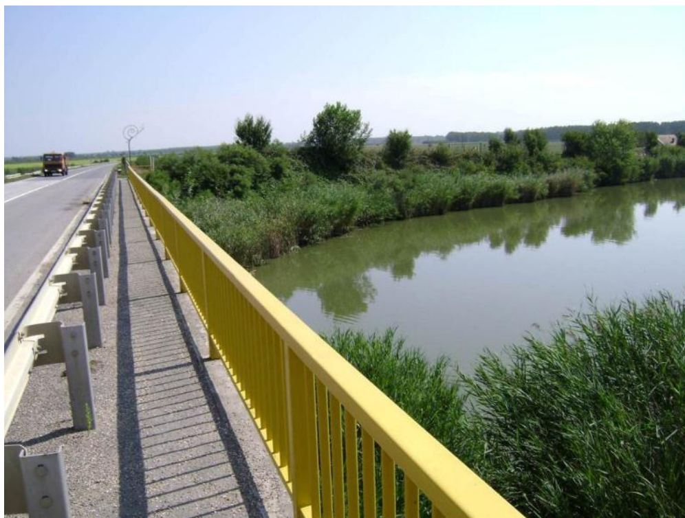
Figure 3.12: Bridge over Jegricka River
