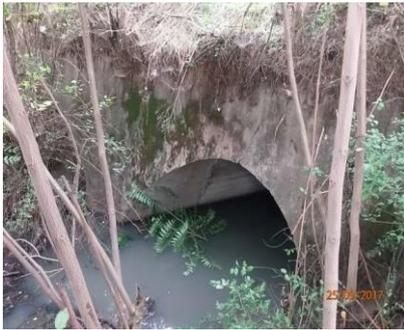
*Figure 6 Solid-headed culvert at km 67+845*
