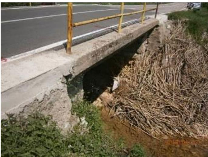
*Figure 9: The box culvert over the Linovstica River*
