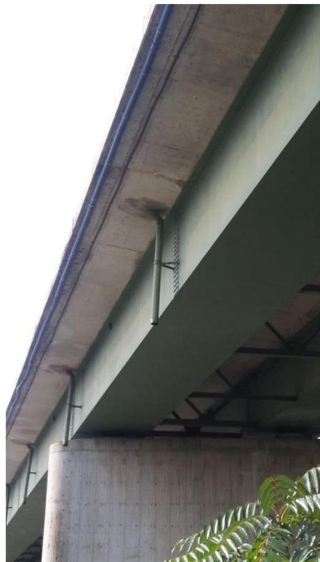
*Figure 18 and 19. The bridge drains*
