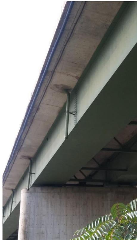
*Figure 18 and 19. The bridge drains*
