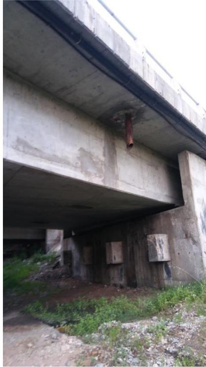
*Figure 16. The bridge drains*
