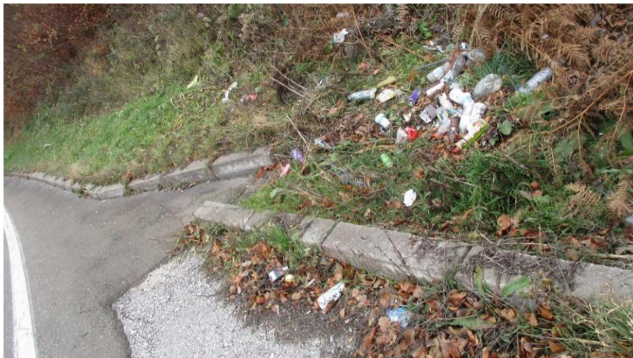
Picture 19. Waste at the outlet of the gutter
