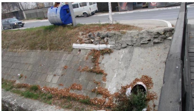
Picture 17. Outflow of drains and collectors into the river Josanica
