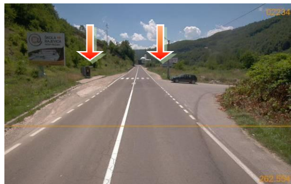
Picture 9. Bus stop at km 262+580 left (unpaved) and at km 262+605 right (unbuilt)
