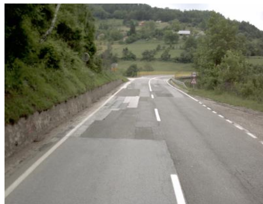
Picture 22. Damage of pavement
