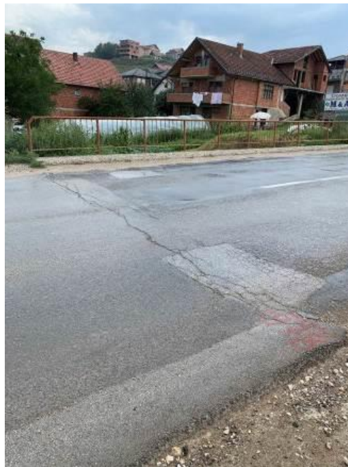
Picture 3. Poor condition of pavement and pedestrian path on the bridge
