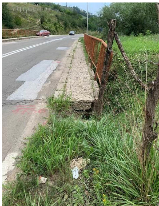
Picture 4. Poor condition of pavement, pedestrian path and fences on the bridge
