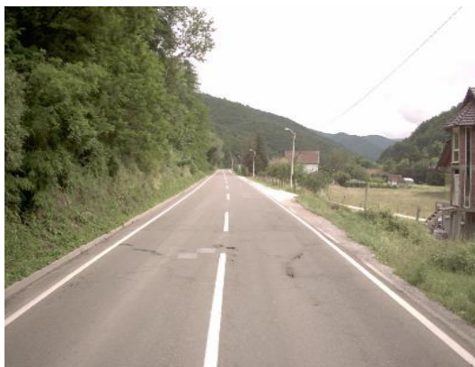
Picture 21. Damage of pavement
