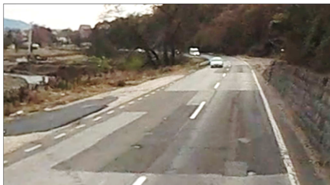
Picture 42. Damage of pavement
