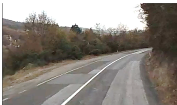
Picture 40. Damage of pavement
