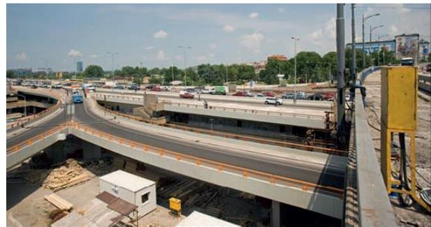
its structure. One, if not the most interesting thing are boxes within the bridge base, at the height of 12m. Most workers perform their work in these boxes although their height is only 1.20m. Gazela bridge consists of 31 parts and each of them hides a team of builders.
