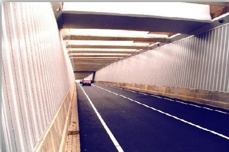
**Figure 5: Visited construction with aluminium absorbing panels in Brunssum.**
