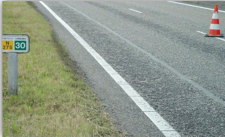
Figure 2: Ravelling probably due to too high porosity.
